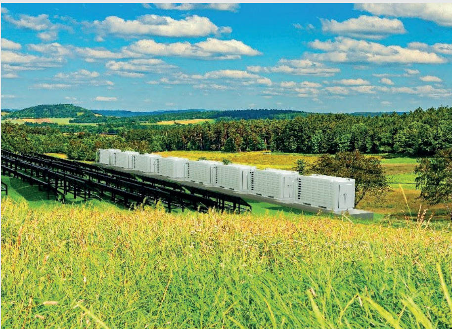
Figure 4 – Typical BESS installation supporting a solar farm
