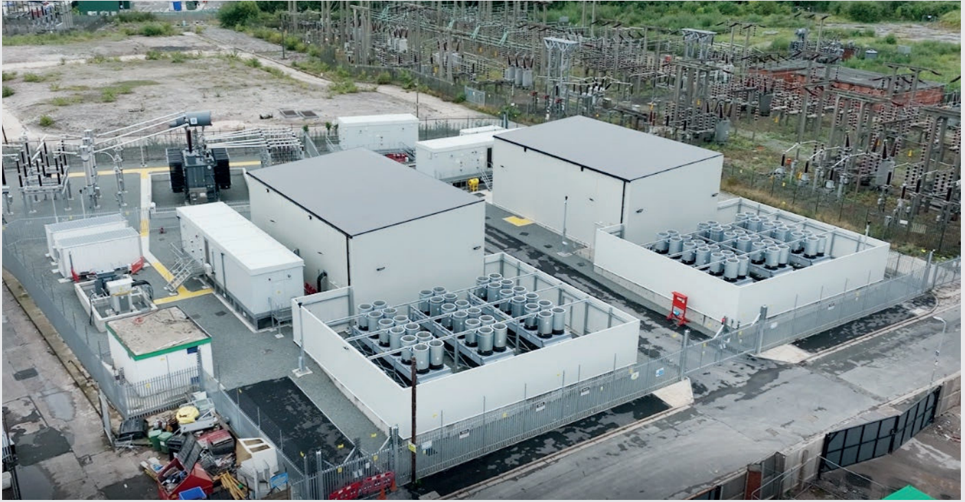
Figure 3 – Lister Drive is the world's first application of ABB's high-inertia SC configuration – housed in the two gray buildings.
